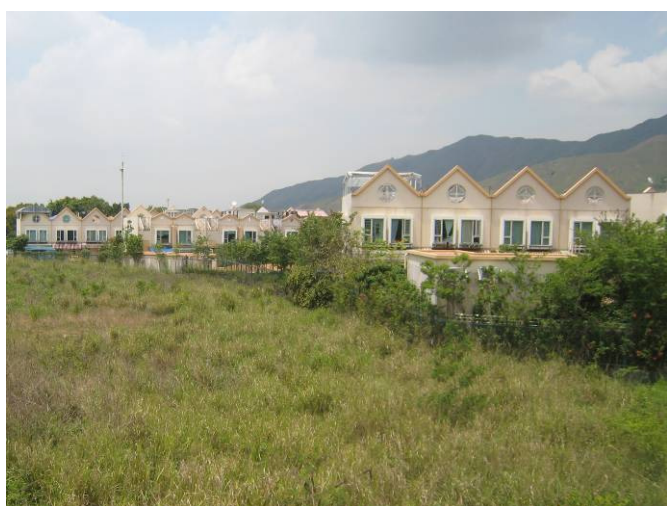
NSR N12. Low-rise residential building, 136, Season Villas
