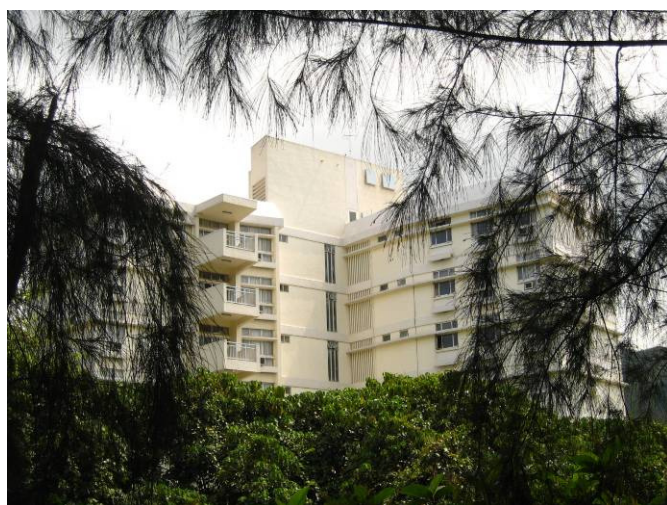
NSR N46. Cheung Chau Court
