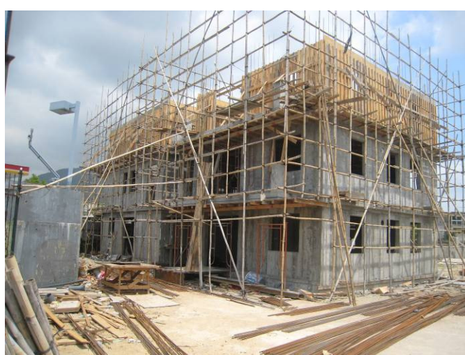
NSR N27. Village house near Petrol Station (under construction)
