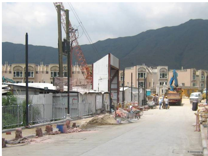
NSR N5. Residential development near Kiu Tau Tsuen (under construction)
