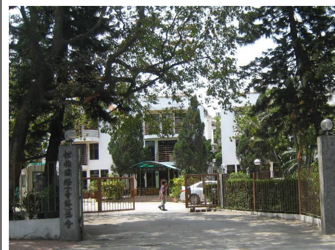
NSR N32. Block 9, Evergreen International Hong
