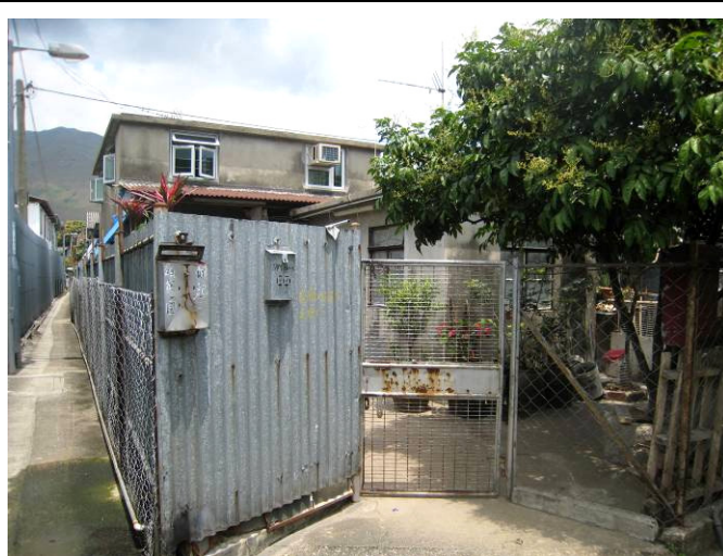
NSR N18. Village house, Chung Ying Yuen
