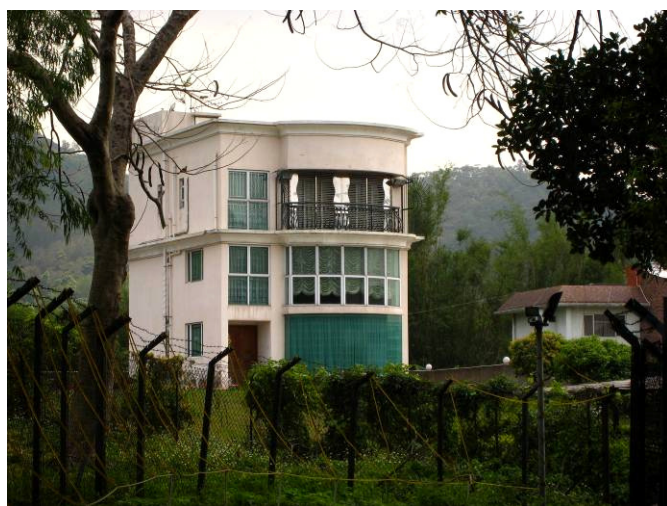
NSR N44. Village house near Route Twisk
