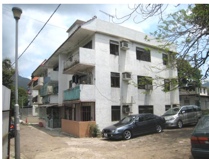
NSR N25. Village house, 28A – 28B, Wang Toi Shan Yau Uk Tsuen
